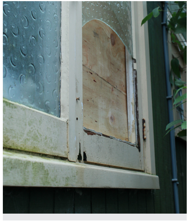
Above left: The kitchen and main living areas had plastic roof sheets with no insulation Above right: Windows in the home were broken and putty was coming away from the rotting timber window frames
