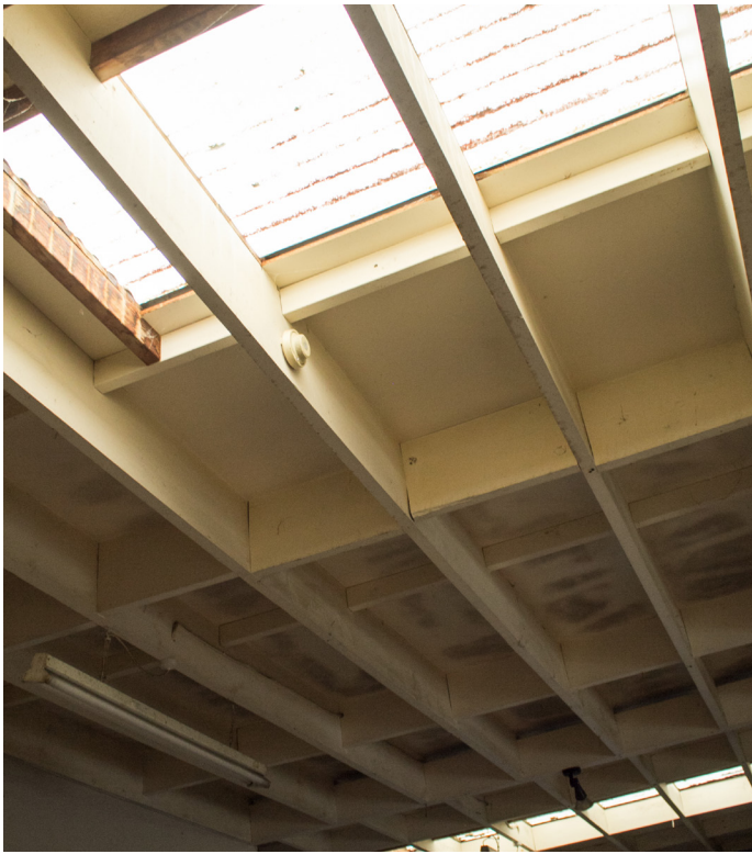
Above left: The kitchen and main living areas had plastic roof sheets with no insulation Above right: Windows in the home were broken and putty was coming away from the rotting timber window frames
